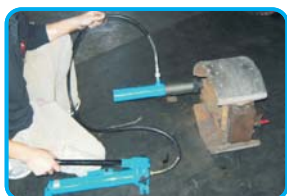
2. To remove anchor pin from brake by hydraulic hand pump. 以手動幫浦施力，將插銷由來令片中拔出。
