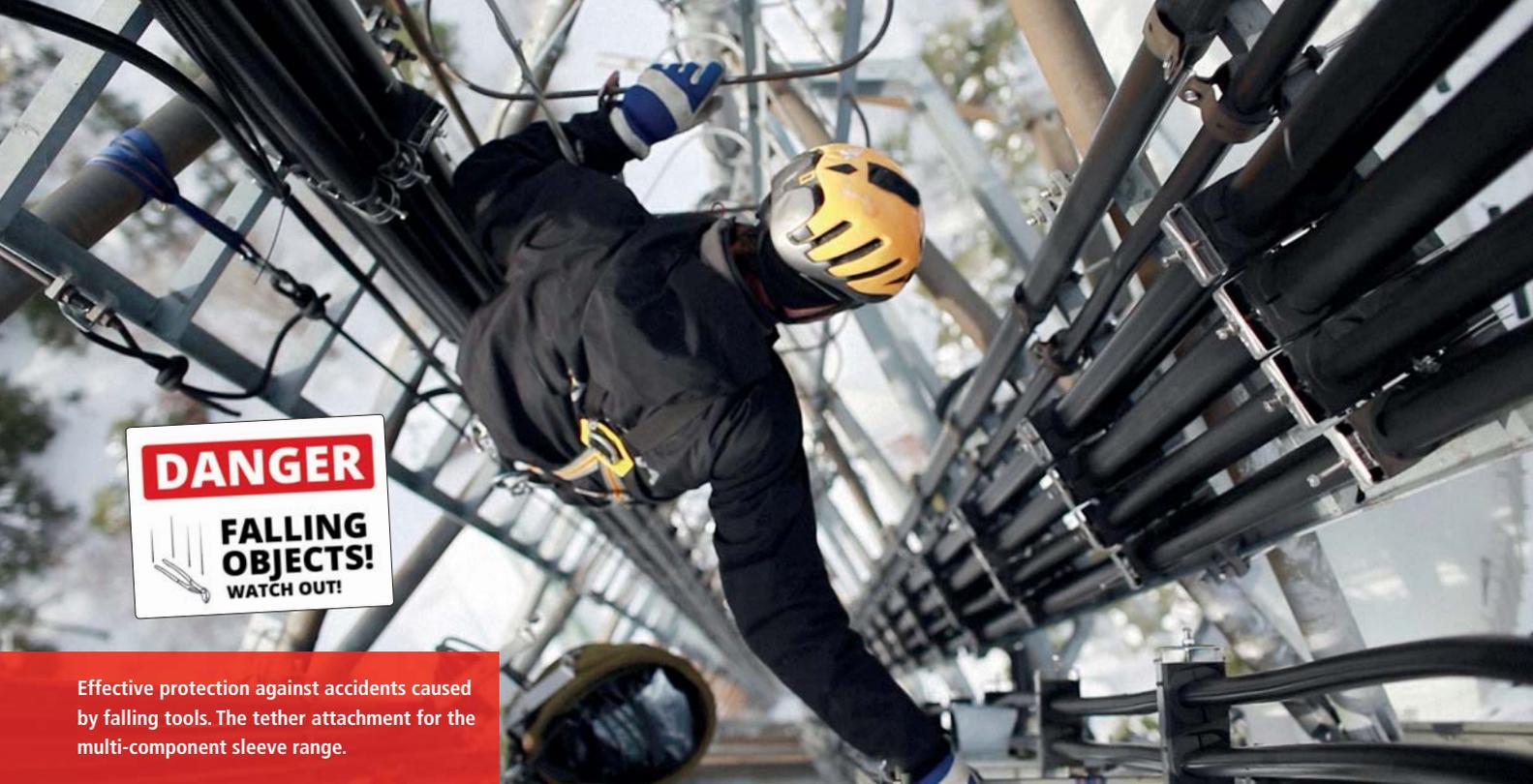
Effective protection against accidents caused by falling tools. The tether attachment for the multi-component sleeve range.
